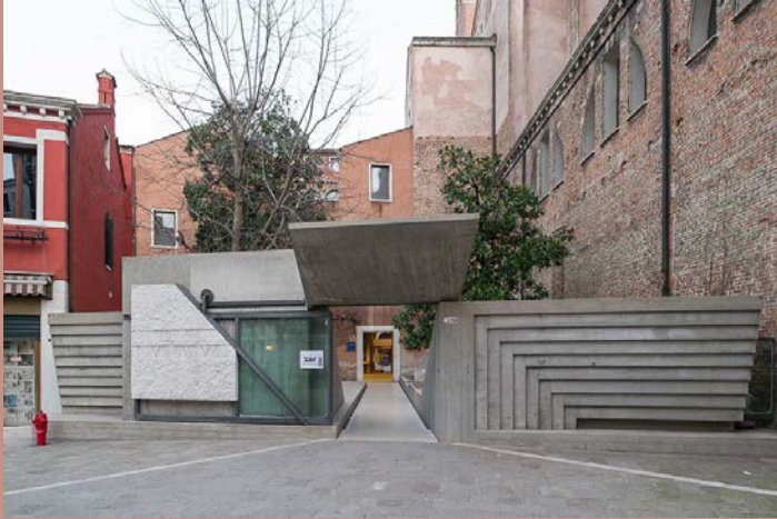
Main entrance of Tolentini. Project design by Carlo Scarpa.
