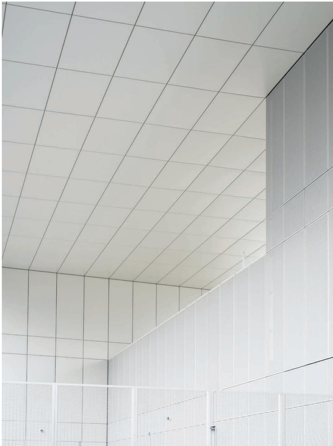
LAN, Quartier de Semi-Liberté, Nanterre. Dettaglio del rivestimento in pannelli metallici bianchi | Detail of the white metal panel cladding. Ph. Cyrille Weiner, 2019.
