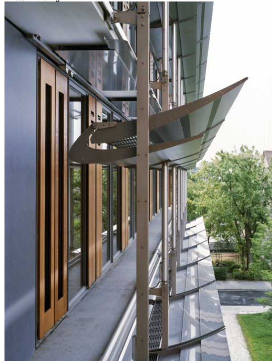
Daylight reflector with light - shelf - effect
